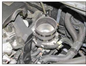
18. Install the provided silicon hose (08434) onto the throttle body and secure with the provided hose clamp.
